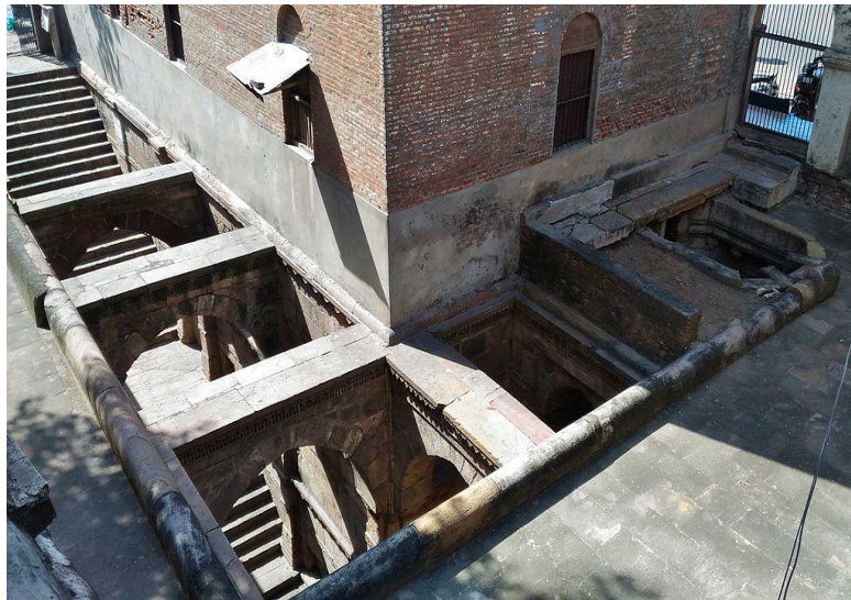
Figure 15 :Right angled construction of step well
