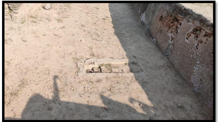
Fig 12: the underground drainage at acropolis.
