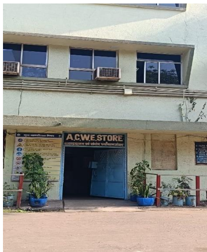
Figure 19 ACWE STORE Entrance
