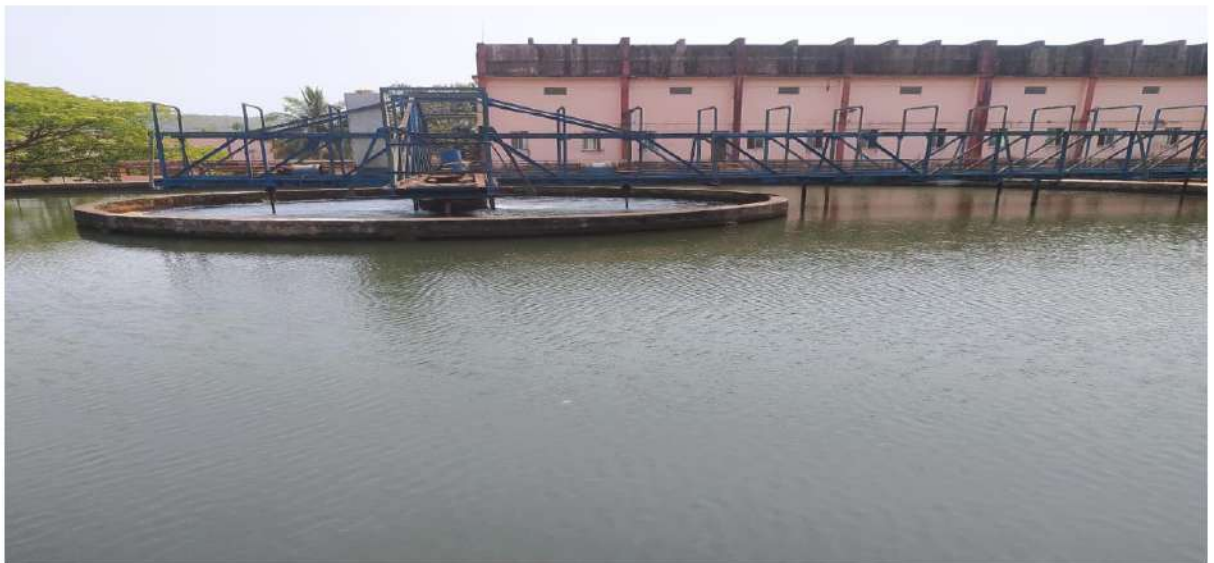
3.10: Sedimentation tank and clariflocculator
