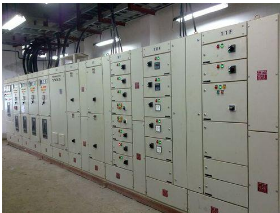
Figure 5 Motor control center
