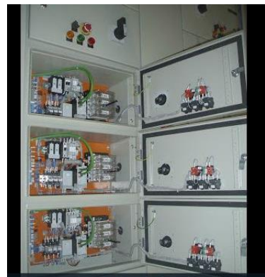
Figure 4 DG control Panel
