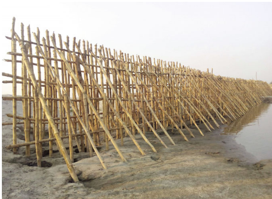
Fig. 12.4 Construction of bandalling. Photograph credit Bokhtiar Hossain Shishir
