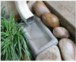
Setting up a splash block is a great idea to divert the flowing rainwater away from the structures foundation. It is a piece of concrete or plastic of a roughly rectangular shape, and is placed below the downspouts that carries rainwater from the roof of the house during rainfall. It absorbs the force of the water that is getting diverted from the roof, and also prevents holes from being dug in the garden due to the eroding force of the pouring water.
