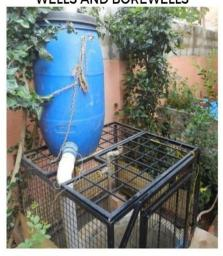
Rooftop rainwater is led through pipes with filter at the end to open dug wells for replenishing underground aquifers. A recharge pit for borewells is a good idea as it pushes back the surface water to the groundwater system. Usually a recharge pit is 1 metre in diameter and 6 metres deep, lined with concrete rings having perforations. These perforations let filtered and desilted water seep from the sides increasing groundwater table.
