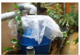
The easiest way to harvest rain is through a rain barrel (make your own from large trash can or an old drum) linked to a pipe fitted to collect rainwater from the rooftop and verandah of the house. To prevent the barrel from becoming a mosquito breeding ground, fasten a tight fitting top to it and screen the ends of the downspouts leading into the barrels. Or simply add a tablespoon of vegetable oil to the stored rainwater. It coats the waters surface and kills larvae by depriving them of oxygen
