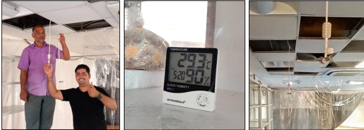
Fig. 7. Installation of the irrigation system and hygrometer
