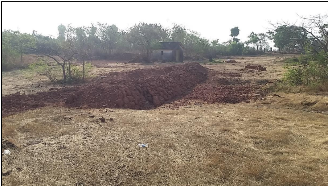
Figure 6.9 : Water harvesting bandhara(bandh) implemented. (Front view)
