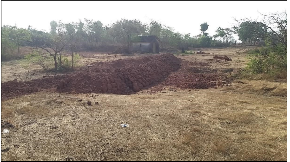
Figure 6.14 : Water harvesting bandhara(bandh) implemented. (Front view)
