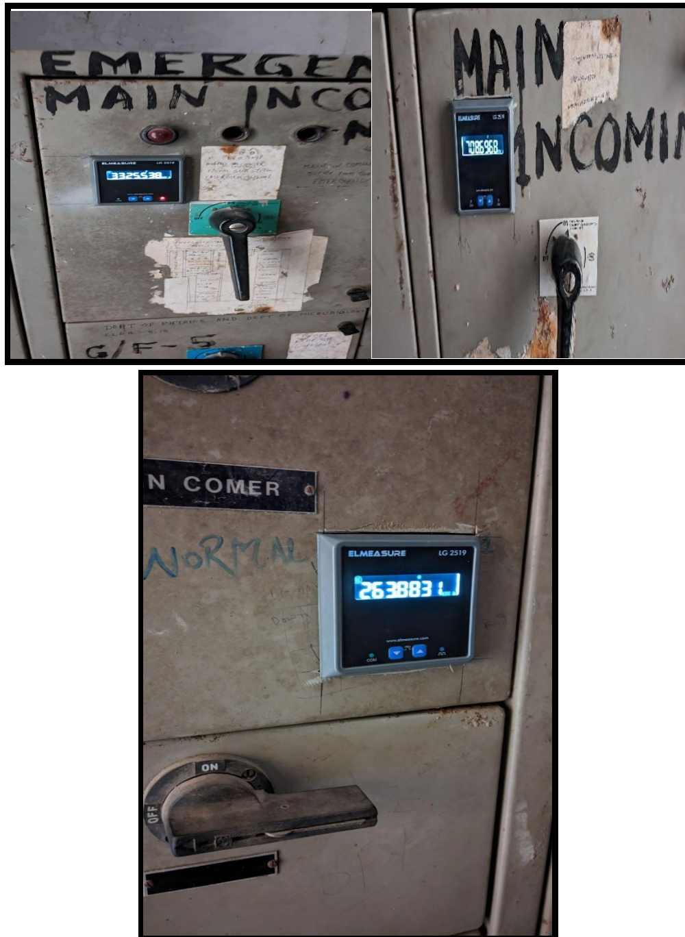
Fig 8.3 Local energy meters fitted for electricity consumption monitoring (2 meters are installed in Block A, 1 meter is installed in Block B)
