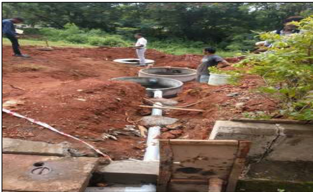
Figure 6.8 : Installations of Siltation, Filtration Chamber and Borewell Pits
