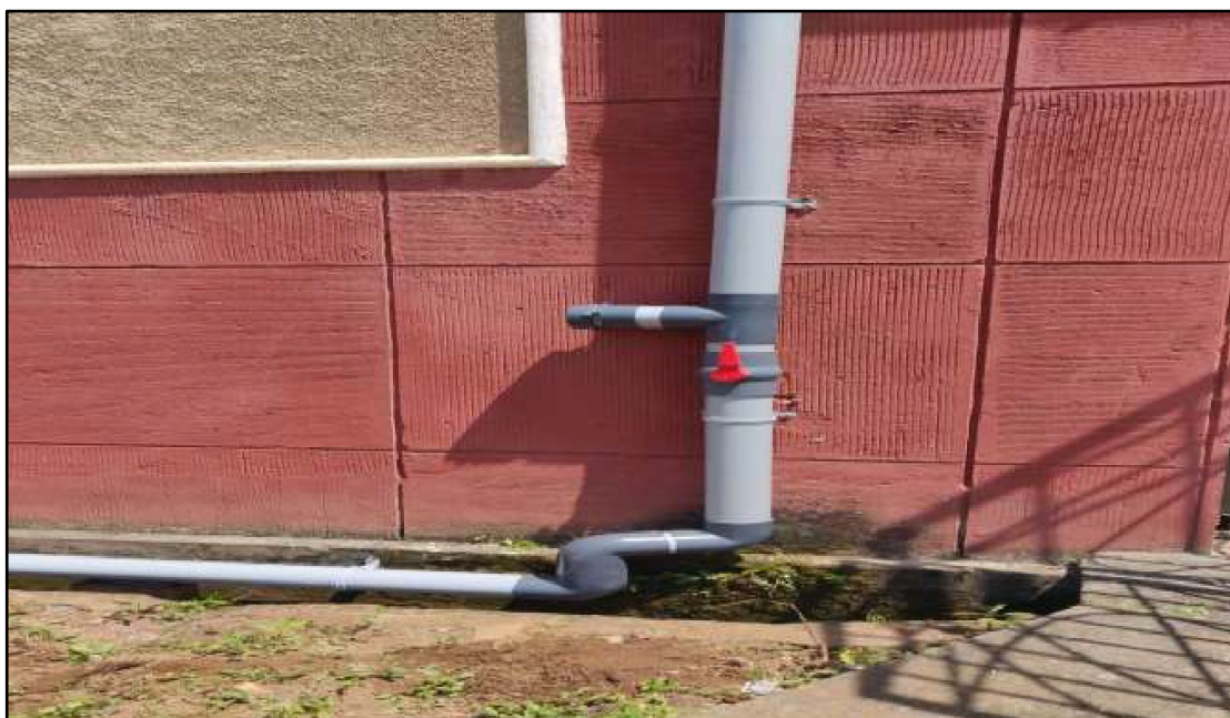
Figure 6.11: School of Chemical Science building under rainwater harvesting piping Connections from Roof for downtakes
