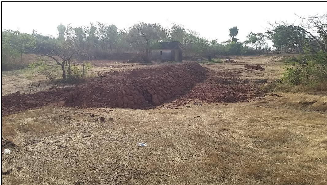
Figure 6.9 : Water harvesting bandhara(bandh) implemented. (Front view)
